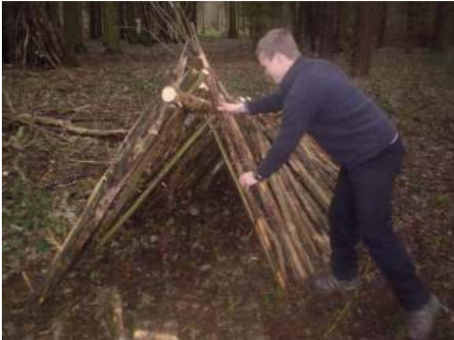
A thermal A frame shelter under construction, a strong green wood frame allows a considerable weight of dead wood from the forest floor to be used to build up the walls of the shelter before leaf litter can be stacked to a depth of 1-2 feet. This kind of shelter will keep you warm even without a sleeping bag if you fill the inside with dry leaves or grass.
